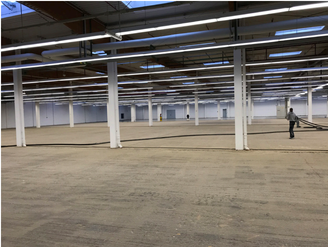
Prepared substrate
