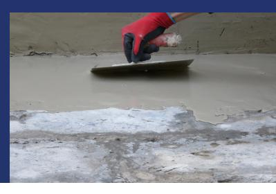
water very fast reducing or completely eliminating the need for water curing and protection. VELOSIT RM 224 creates an extremely well bonded, rigid, abrasion resistant layer on the substrate.
