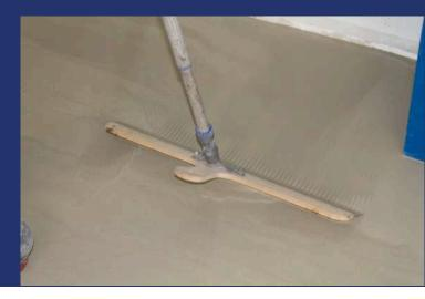
VELOSIT SL 501 surpasses the requirements of EN 1504-3 class R2 for concrete repair (CR) and can be used according to the principles 3 and 7 acc. to EN 1504-9.
